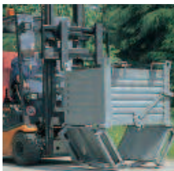
2. base being closed with the aid of steel roller
